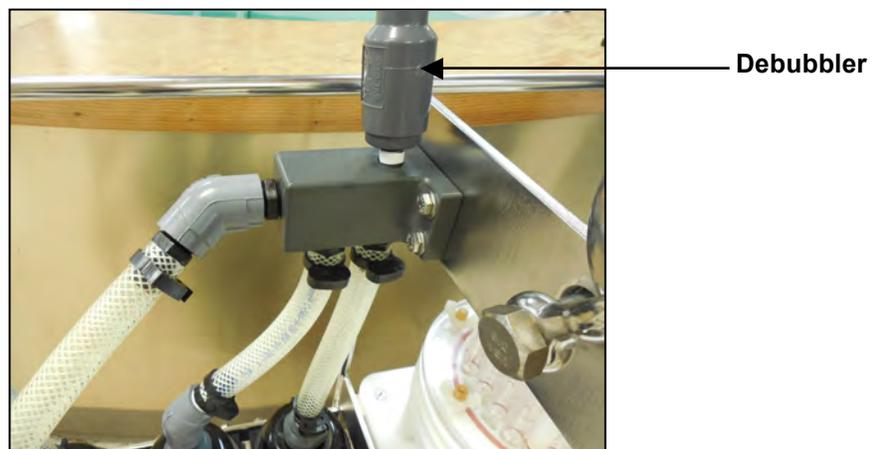
*Figure C.1.3-2: Screw Debubbler into Manifold*
